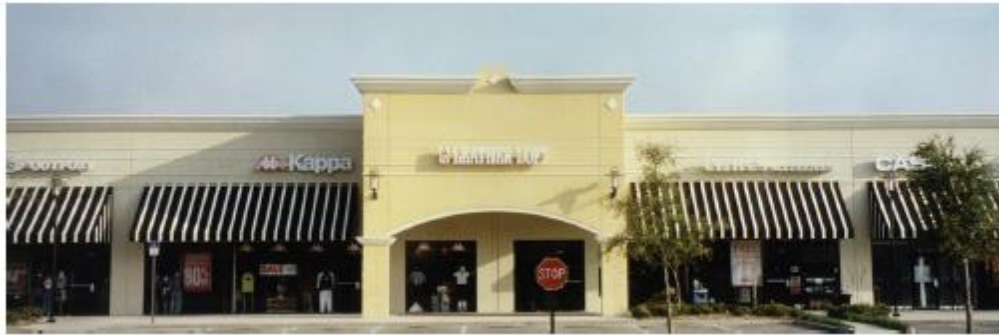
Figure 27. Example Building Entrance Enhancement
